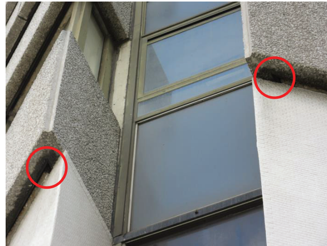
Photograph 2 Crevices underneath concrete blocks on Building 1.
